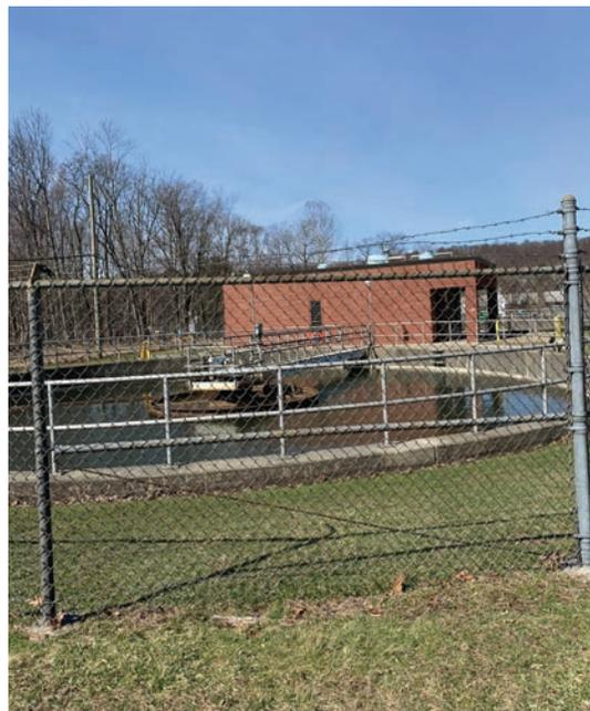
The facility is also subject to flooding from the Peckman River during significant rain events. Portions of the property are located in the official FEMA flood maps. In addition to flood damage, the facility also experiences problems with capacity during significant rain events as some of the facility's inflow connections are from sources that should not go to the facility. For example, sump pumps in homes connect to the facility rather than to catch basins or the street.
